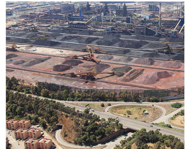
Residential buildings in the district Tamburi and ILVA mineral park deposits lie 130 meters away from each other.
