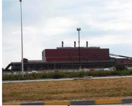
Steel production plant
