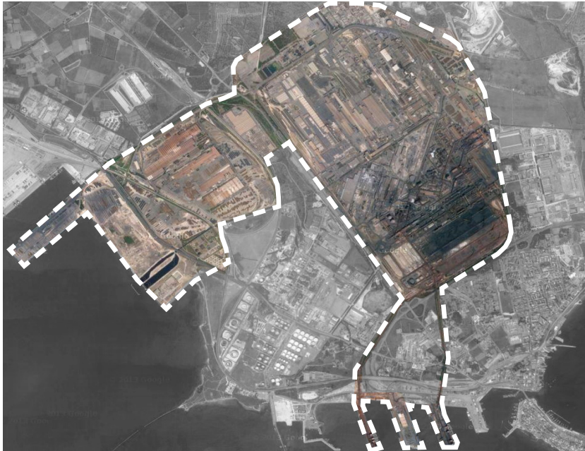
ILVA, with its surface of about 15 km 2 , is the biggest steel production plant in Europe.
