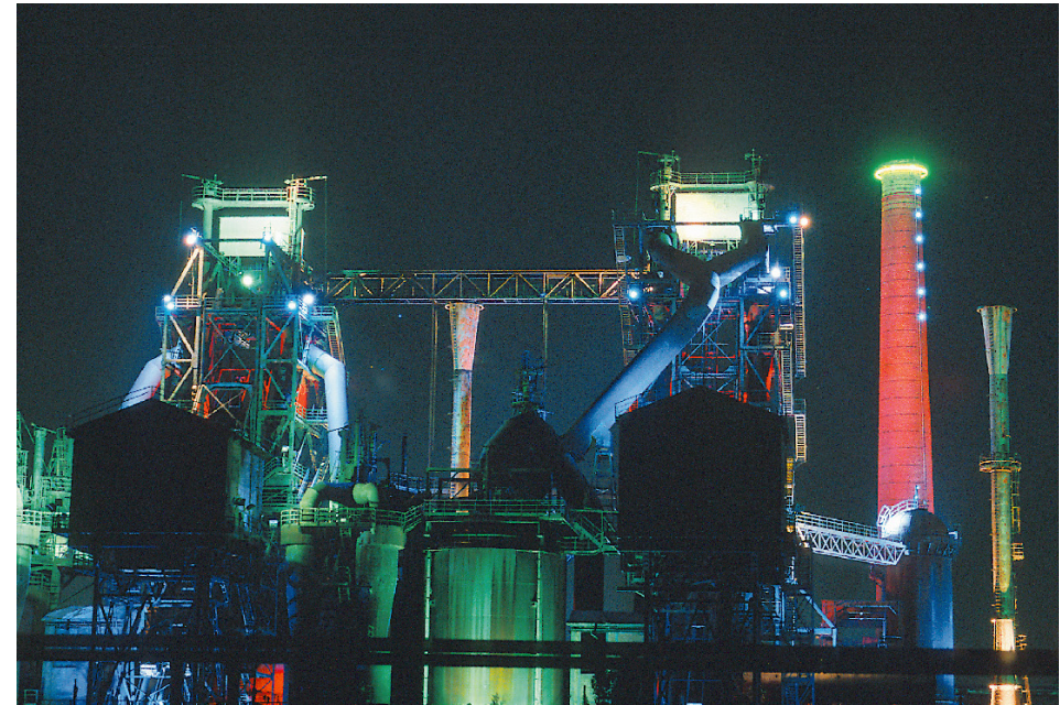
Jonathan Park's lighting concept for the Blast furnaces in Duisburg-Nord park.
