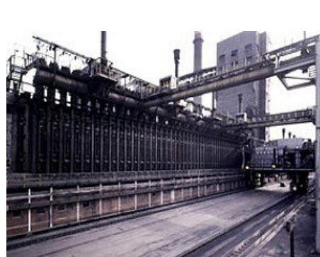
Coke ovens area
