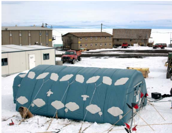
Fig. 1: Inflatable habitat deployed in McMurdo station, Antarctica. Credit: Peter Rejcek.
