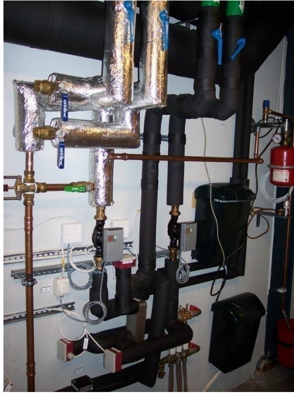
Figure 13. Photograph of the valve group from figure 12.
