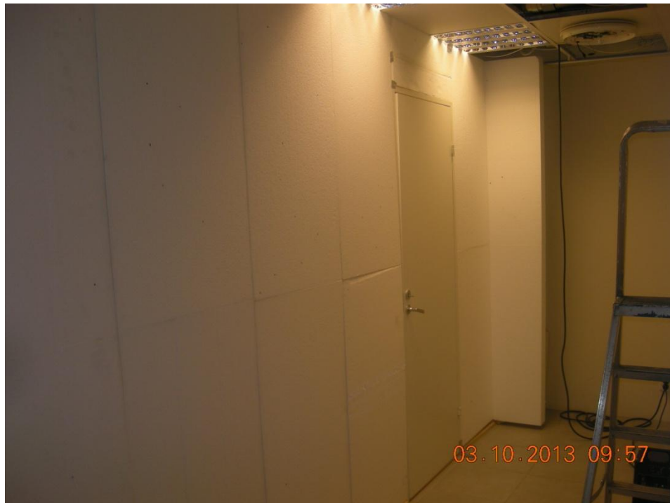
Figure 20. Photograph illustrating the right temporary Styrofoam wall in figure 19, which was shared by the two considered spaces and had a built-in door.
