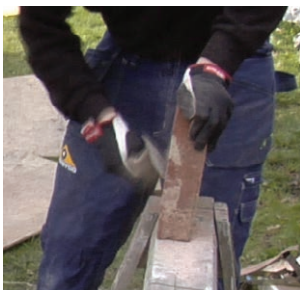
The bricks had to be cleaned to ensure a good adhesion with the mortar. Then dried for the same reason and to make them as light as possible, although only a few of them were of the light weight type made by mixing in saw dust in the clay.
