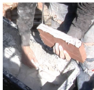
Although several options that automated the laser movement were tested, it was found to be easiest when it moved on command, which in this case meant someone sitting by the computer. Only then the mortar could be applied, called "Lareado" in Catalonia.
