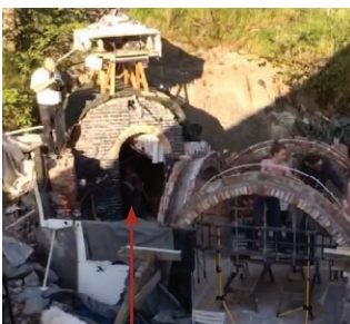
Although several options that automated the laser movement were tested, it was found to be easiest when it moved on command, which in this case meant someone sitting by the computer. Only then the mortar could be applied, called "Lareado" in Catalonia.
