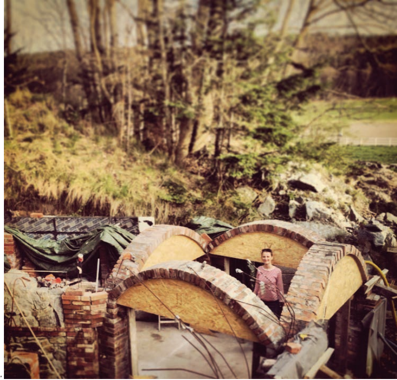
The arches were erected on the form work.
