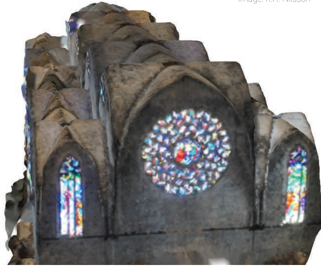
The ceiling of Santa Maria del Mar, viewed from the outside. Roughly the same geometry is reflected on the exterior roof. Here, the scanned point cloud has been converted into a mesh surface with good results.
