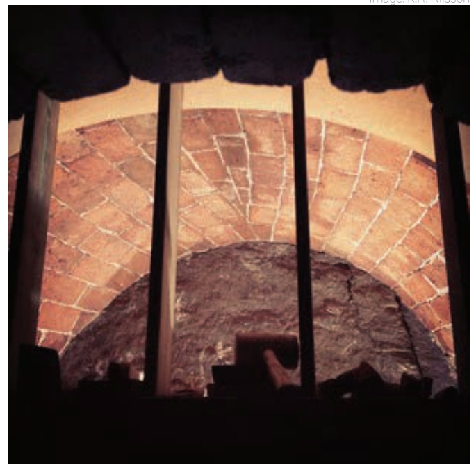
A picture of the first vault constructed during the experiments. The pattern has a resemblance to patterns seen on wooden ship hulls.
