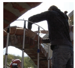
The tile was aligned in accordance to the laser and put in place, letting go a few seconds later as the mortar dried and held the tile in place.
