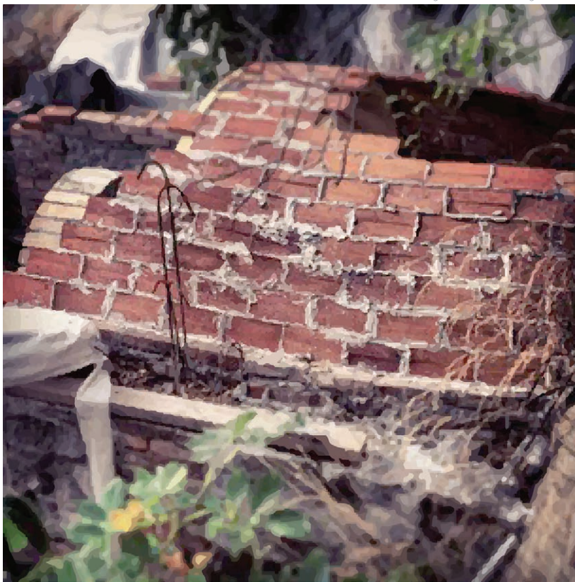
The first course of the first tile vault under construction at the test site, using 2.5 cm thick brick tiles made from recycled old bricks and fast setting plaster of Paris (gypsum mortar).
