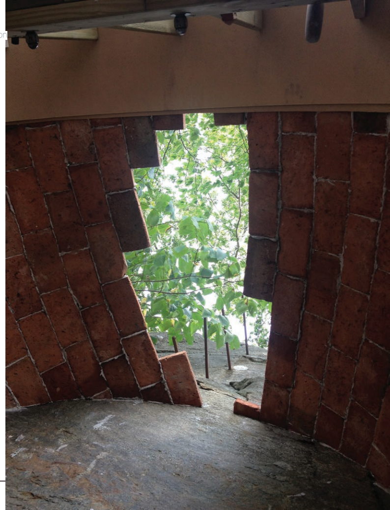
Image of the almost finished vault showing the adaptable form work in the top, the simplicity of the details. But this was also the area which had the lowest quality of the curvature.
