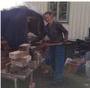
A lot of pre work had to be done. The tiles were salvaged from a refurbishment in an old house in Gothenburg and some from a demolished 19th century service building (Swedish: brygghus) and brought in by truck. All bricks were then cut into tiles.
