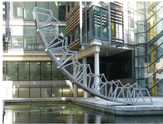
Figure 4.5: The Rolling Bridge in London, example of a collapsible bridge. (in Wikimedia Commons, the free media repository, Retrieved 2014-08-08 from: http://commons.wikimedia.org/wiki/File:The_Rolling_Bridge_by_Thomas_Heatherwick,_Paddington_Basin2.jpg )
