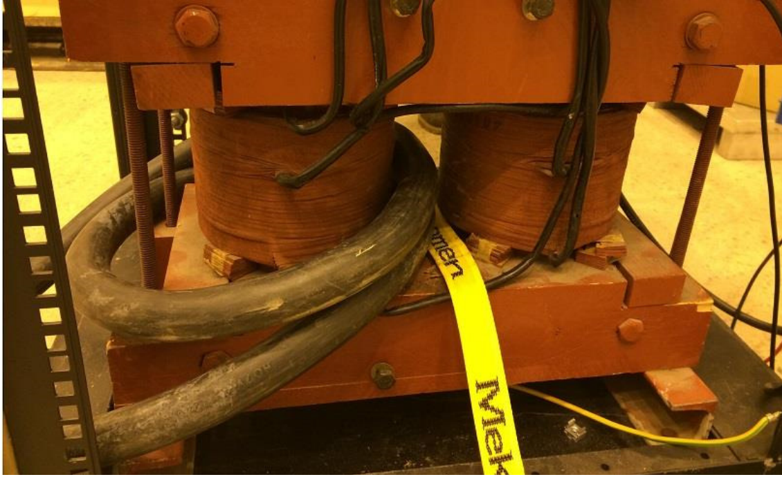
Figure 3.19 Transformer secondary winding of impedance measurement.
