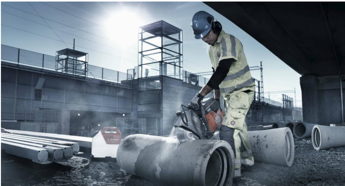
Figure 1.2. A concrete cutting professional using a K760 to cut a water pipe (Husqvarna Construction AB, 2014 A)
