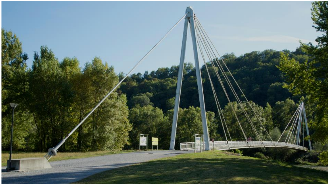
Figure 44. The Laroin footbridge in France. The CFRP cables that are supporting the span can clearly be seen together with one of the steel cables that anchor the bridge on the sides (geocaching.com, 2014).
