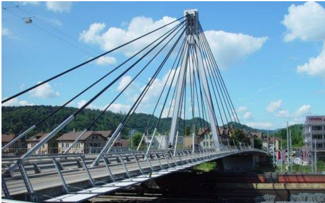
Figure 42. The Stork Bridge in Winterthur, Switzerland (decentlab.com, 2014).
