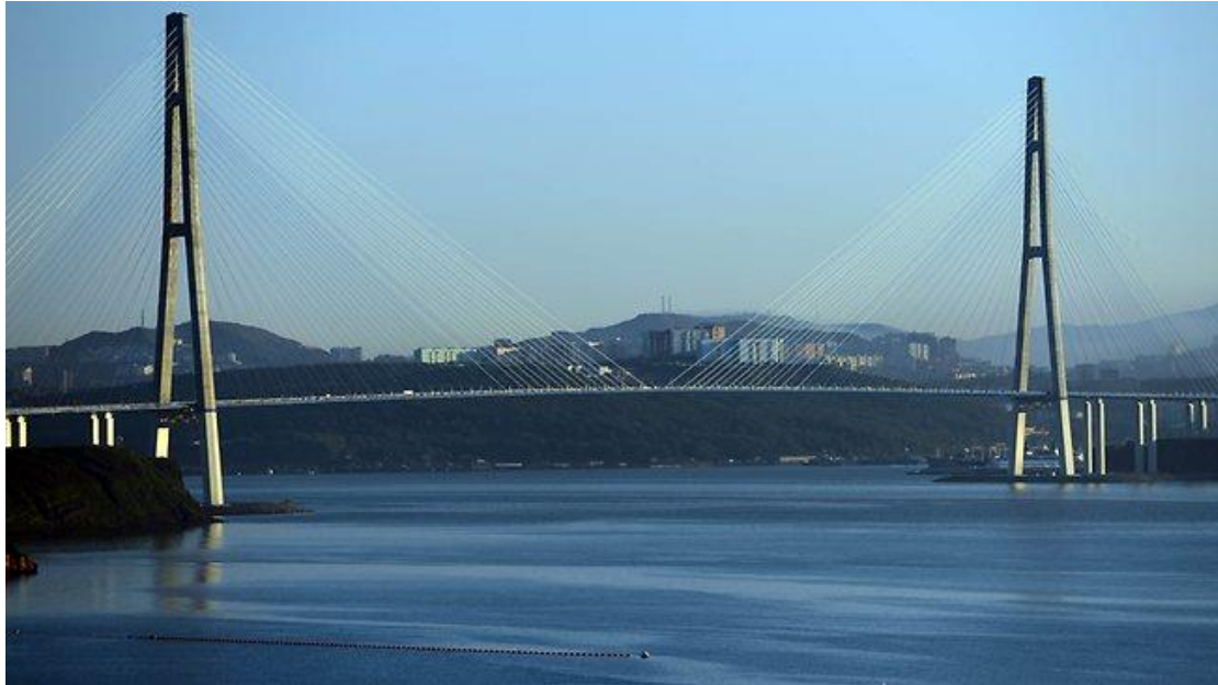
Figure 8. The world's longest cable-stayed bridge, Russky Bridge (1 104 meters), Russia ( news.com.au , 2014).
