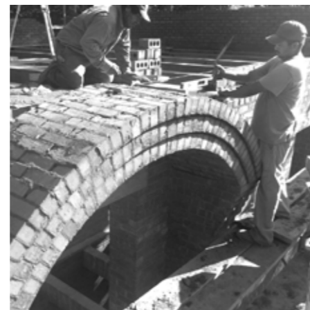
Brick arch construction, Columbus USA
