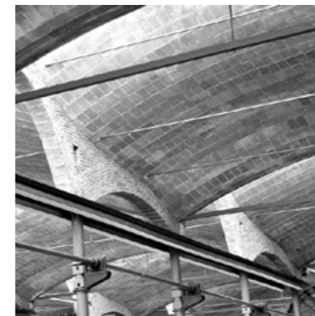
Brick arches and double-curved roof in Vapor Aymerich by Lluís Muncunill, Terrassa Spain 1909
