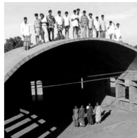
Segmented vault of earth blocks, Auroville India 1995
