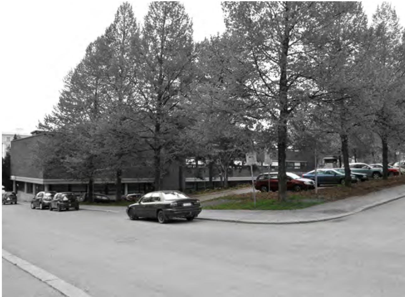
Available building plot for extension.
