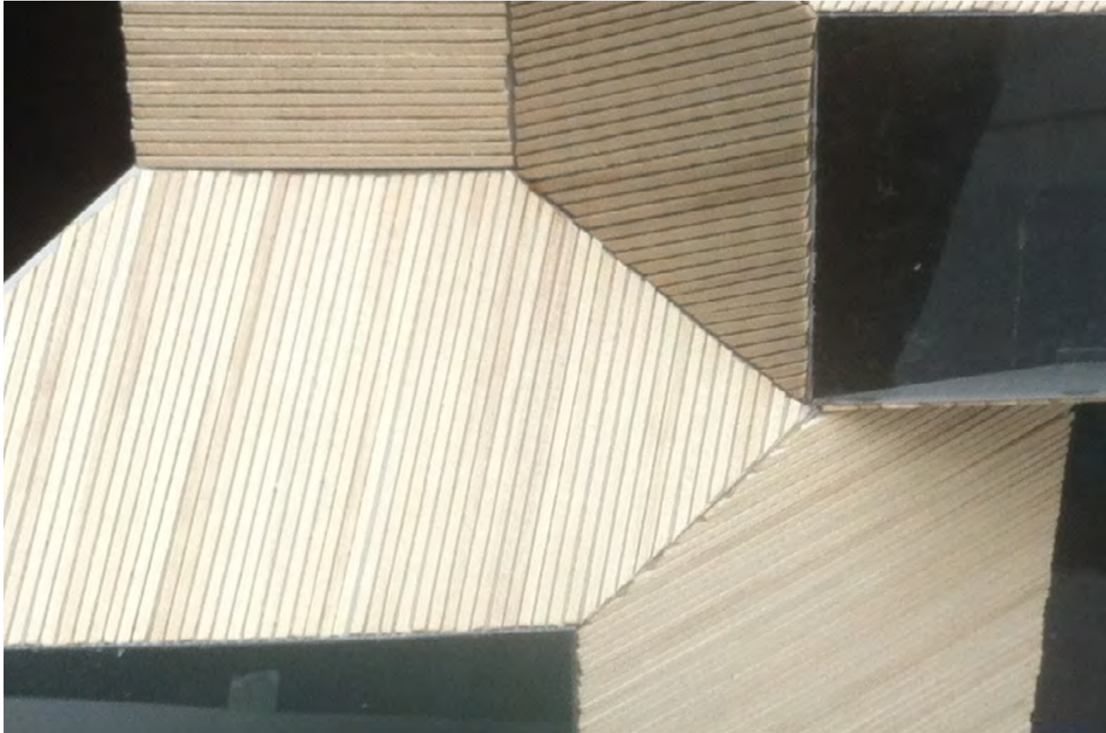
Detail of the meeting between the surfaces of the facade. The wood panels have different directions on each surface.
