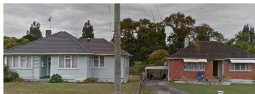
Post war detached state housing. With weatherboard cladding to the left and brick cladding to the right. (Authors own image, 2014)
