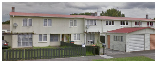
State housing units (1960-1970). Two storey with a mix of vertical and horizontal timber boards with corrugated iron pitched roof. (Authors own image, 2014)
