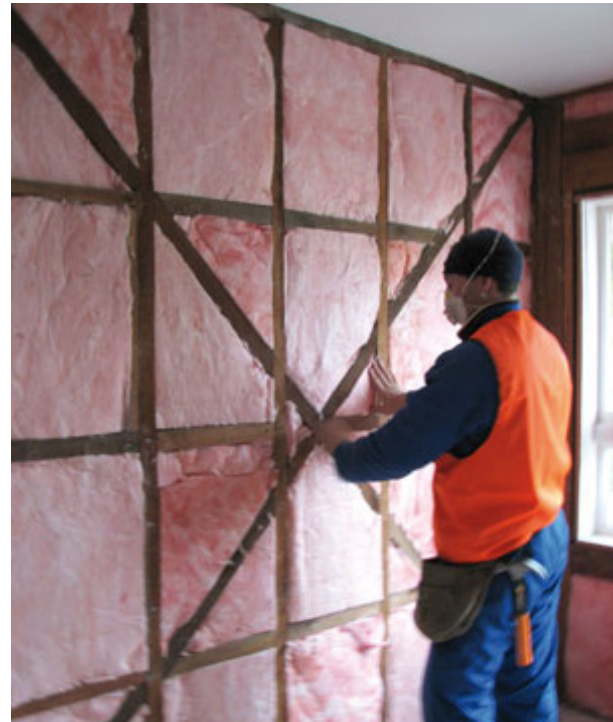
Option 1 - 90mm of Pink Batt insulation installed between timber frames from the interior. R2.4 is achieved.
