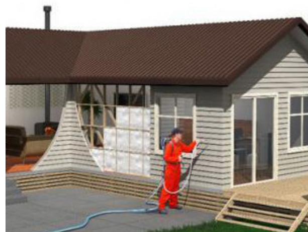
Option 2 - Exterior AIRFOAM Wall Insulation. Timber studs are filled with AIRFOAM via small holes in the exterior cladding.
