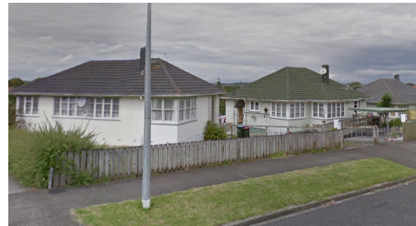
Contemporary photograph of post-war detached state housing (1940-1950) in Glen Innes. Single storey timber weatherboard with hipped tiled roof. (Authors own image, 2014)
