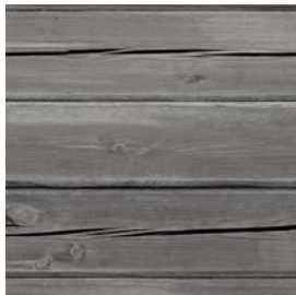
Timber walls Local pine heartwood. Largest dimensions ca. 0,3x0,3x5,5m.
