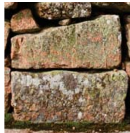
Stone cover in local red granite on foundations and gravel paths
