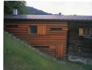
Gugalin House, Switzerland Peter Zumthor (1994) Would a highlighted meeting between new and old create a better understanding of the a place specific identity?
