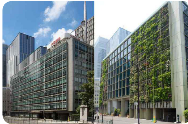
Pasona HQ, a business building located in Tokio, Japan Image source: Inhabitat.com
