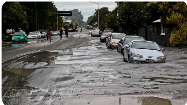
Liquefaction in Kilmore St Source: keithwoodford.wordpress.com
