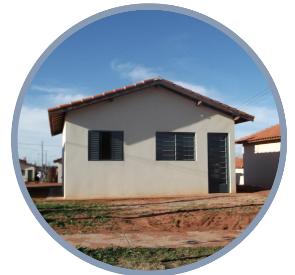
Typical MCMV house
