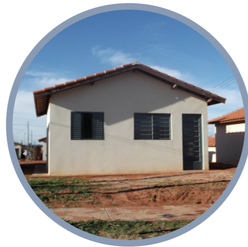
Typical MCMV house
