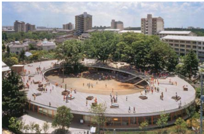
Fuji Kindergarten, Tezuka Architects
