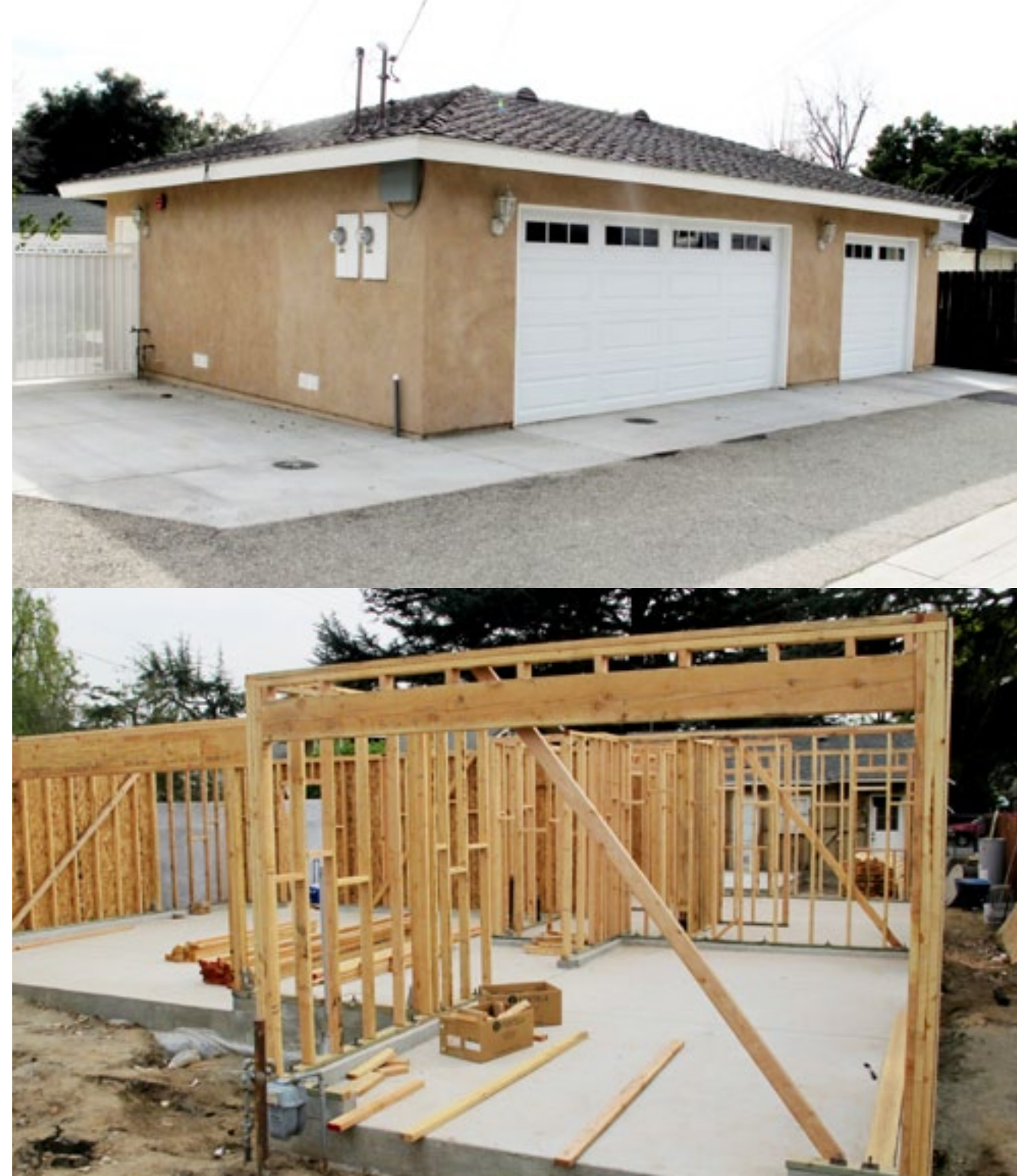
Two La Verne granny flats; one finished and one in the making. They can mostly only be seen from an alley way behind the main building and due to the hard garage requirements, most homeowners combine the granny flat with the garages which make them all look like a three car garage.
