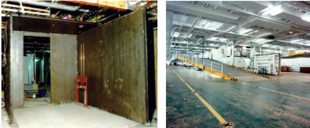
Figure 2.7 Internal walls made of SSP (left), internal ramp of a Ro-Ro ship made of SSP (Kozak J. , 2009)
