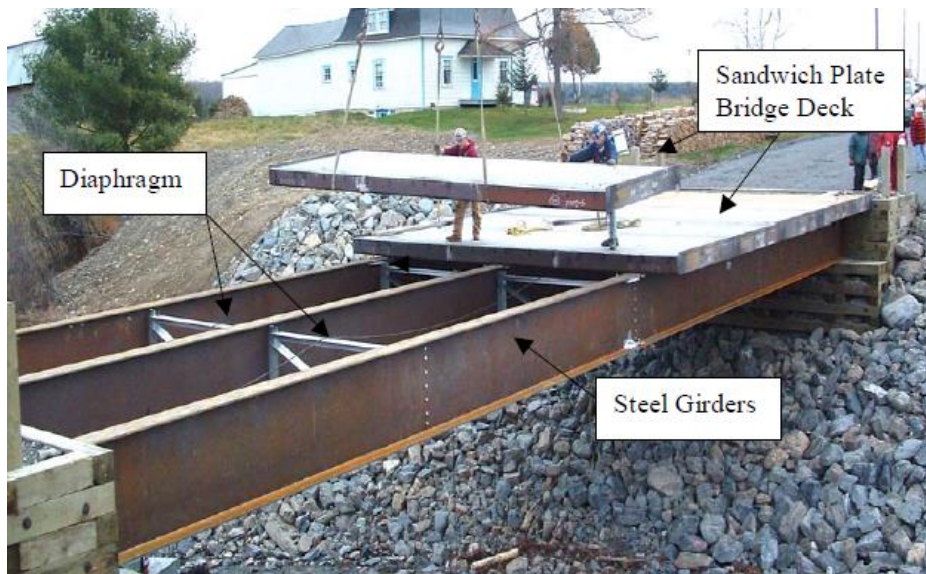
Figure 2.9 The Shenley Bridge (Harris, 2007)
