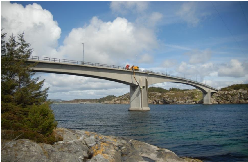
Figure 3.1 Picture of the Bakkasund Bridge. (Photo: Claus K Larsen 2 , 2013)
