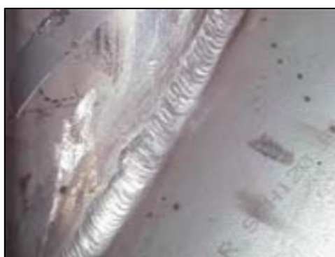
Figure 2.16: Weld after pickling, the tint of has been removed and the corrosion resistance has been restored (Euro Inox, 2004).
