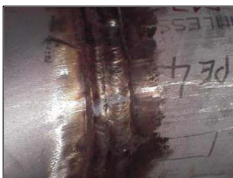
Figure 2.15: Visible weld tint of stainless steel weld. The tint indicates that chromium has reacted and subsequently is depleted at the surface (Euro Inox, 2004).
