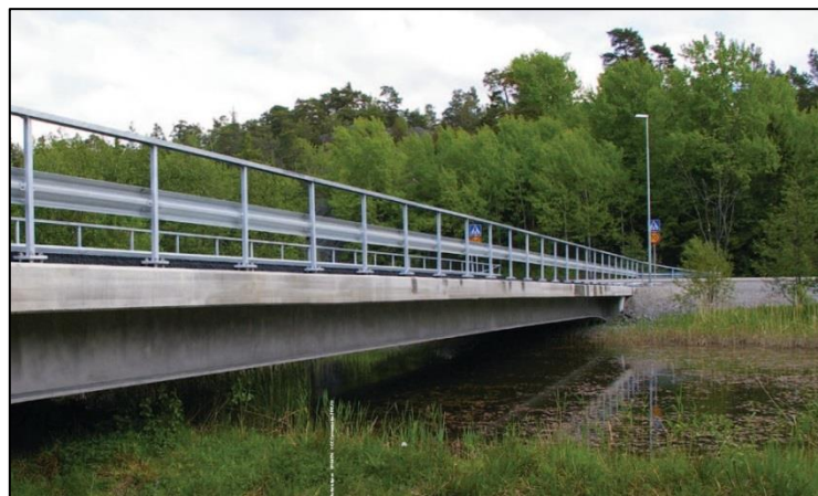
Figure 2.27: Road bridge in Nynäshamn, Sweden. The composite bridge structure consists of two stainless steel I-girders and a reinforced concrete deck (Finnås, 2012).
