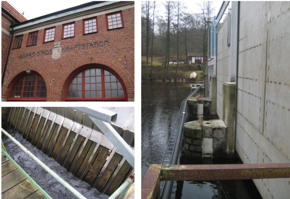
Figure 4.3: Hulta hydropower plant. Upper left: hydropower station, bottom left: cleaning racks at the turbine intake and right: dam construction. (Steinmetz, M., 2014, Hulta hydropower plant [photography])
