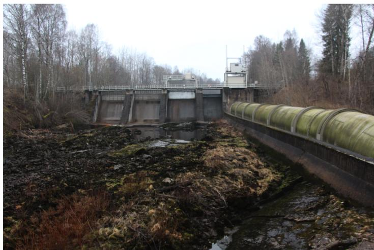
Figure 4.9: Axelfors hydropower plant. Dam construction and tube. Spillways are closed and no water is passing by the turbine. (Seger, F., 2014, Axelfors hydropower plant [photography])
