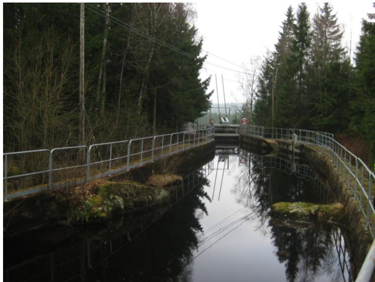
Figure 4.7: Häggårda hydropower plant. Headrace leading to intake to tube. (Steinmetz, M., 2014, Häggårda hydropower plant [photography])
