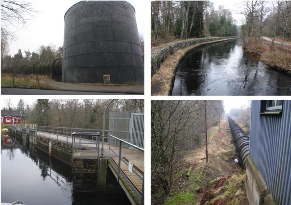
Figure 4.2: Haby hydropower plant. Upper left: the swelling tower, upper right: headrace, bottom left: dam construction and bottom right: tube (Seger, F., 2014, Haby hydropower plant [photography]).
