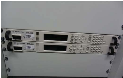
Figur 24: "Befintliga spänningsaggregat (Agilent)"
