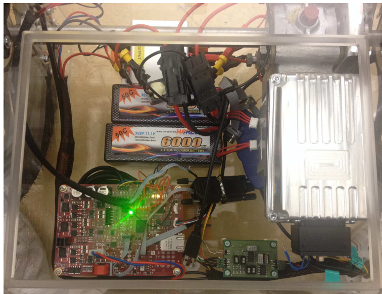
Figure 6.2: In the left bottom corner is the red XMC board, the bottom right is the green SGB board. Inside the metallic box to the right is the motor control board.
