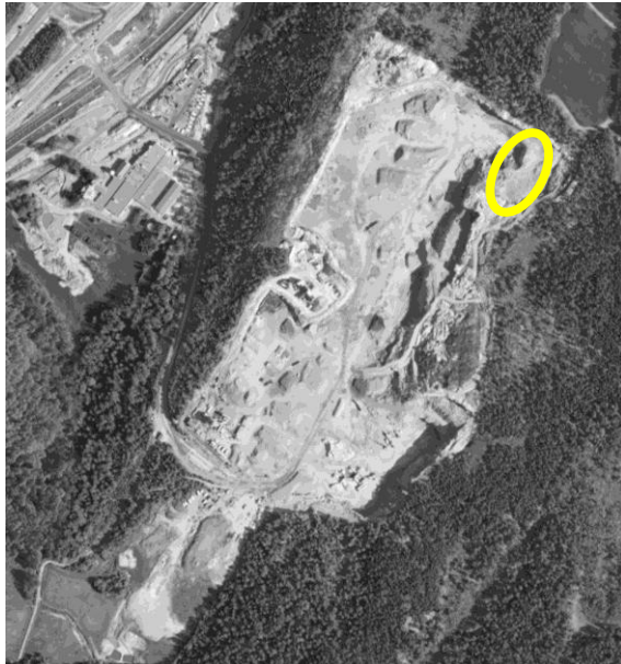
Figure 3.2 Photo of Ale quarry © Lantmäteriet [i2012/1099].
