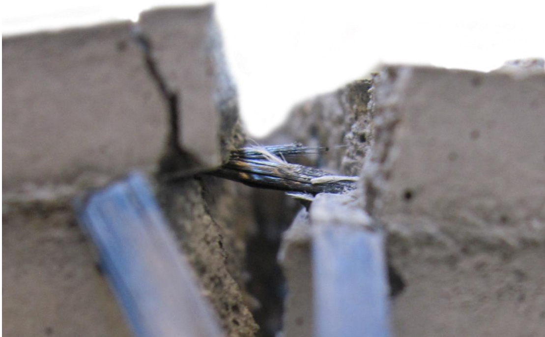
Figure 4-4 Experiment specimen after failure
