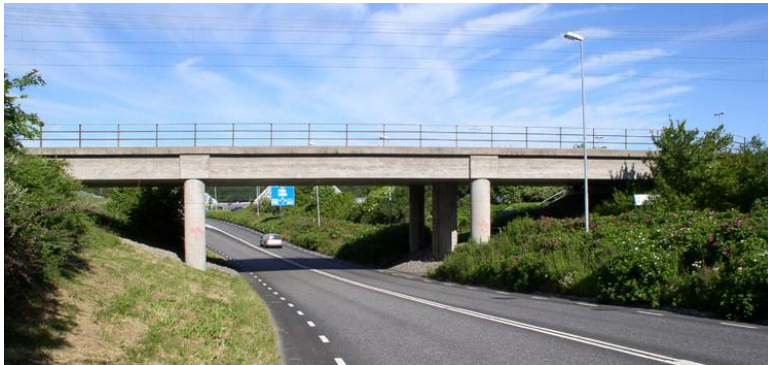
Figur 4. Plattbro i betong (Rutgersson, 2008).
