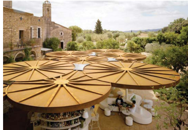
Parasol structure of rusted steel, at Castel d'Emporda, in Girona, Spain. A reference for the parasol roof I propose at the square.
