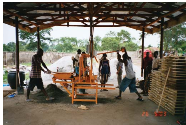
Sustainable brick production, by CIDEM.
