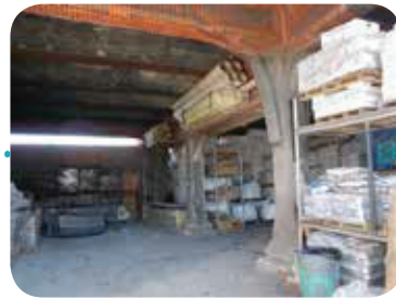
The original concrete columns and beams can be seen indoors. All weather protected spaces are in a good condition.
