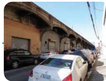
The arches create a rhythm along the facade and give a sense of tradition and familiarity to the building.
