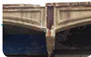
The reinforcements in the arches have become exposed at a few spots where the concrete has fallen off. This has resulted into corrosion.
