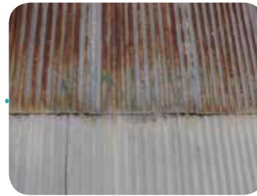
Corrugated iron is used as a facade material in many places. It has become rusted.
