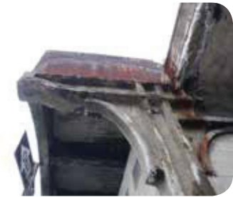
The profiles and joints of the original columns and cantilevered beams are visible at the corners.
