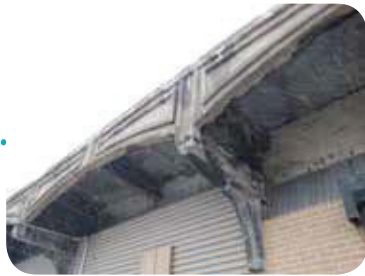
The arches are ornamental pre-cast concrete with steel reinforcements. The arches are supported by cantilevered beams.
