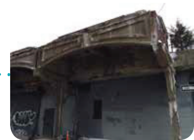
Most of the concrete deterioration is due to a freeze/thaw cycle where moisture in the pores freezes and expands causing cracking and scaling.
