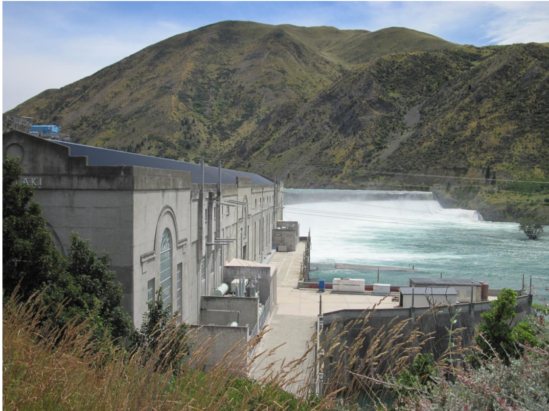
Figure 2.5 Waitaki power station after a rainy period. The station is smaller than the upstream stations and cannot use the energy in the high flow for power generation. On the right in the picture one can see that water is instead spilled past the station without being used.
