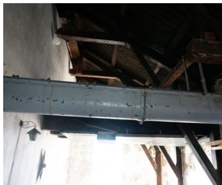
Beer pipe, Storage building
