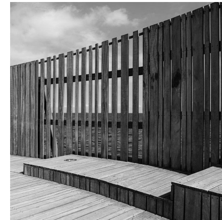
Kastrup, gaps in the board
