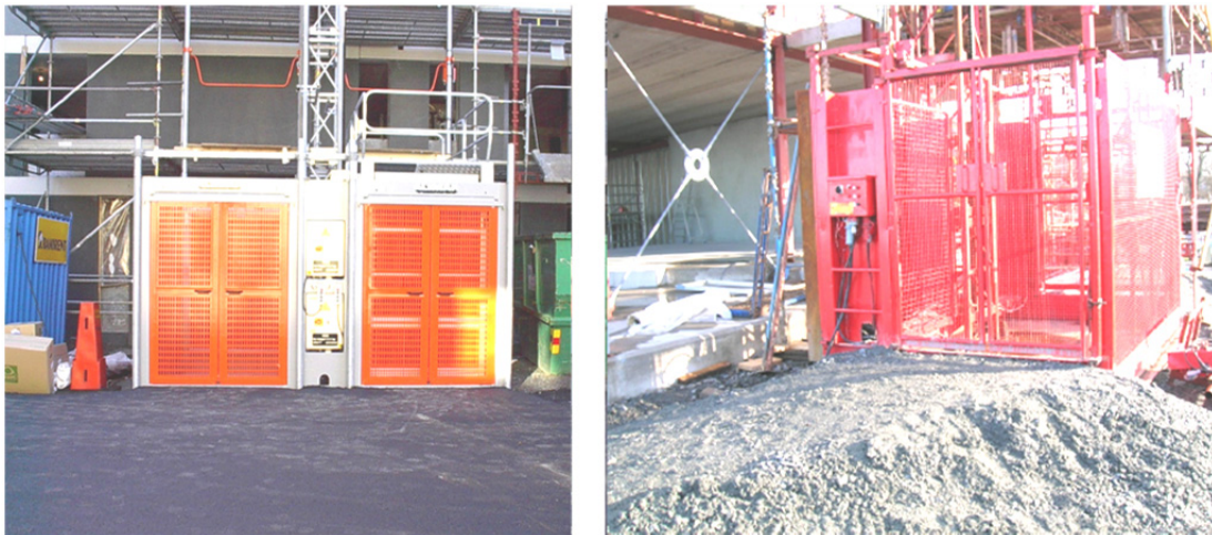
Figure 6.6 Aligned elevators: pallet lifts can be used (Source: Lindén, 2011).
