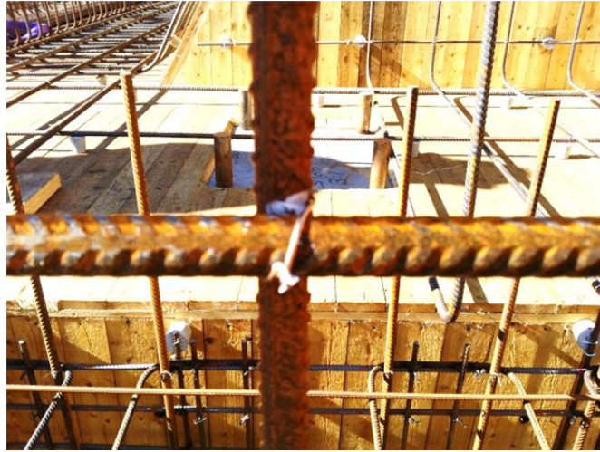
Figure 4.1 Installed reinforcement in casting concrete forms.
