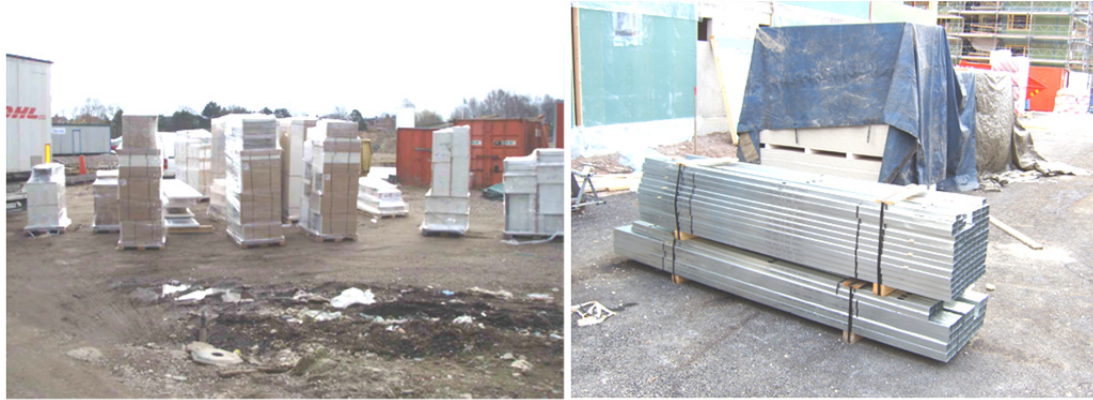
Figure 6.2 Materials storage on site (Source: Lindström and Skude, 2008; Lindén, 2011).
