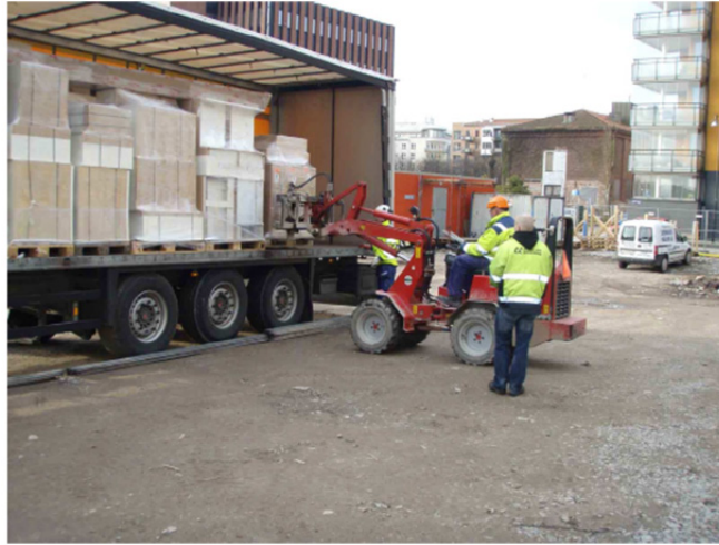
Figure 6.1 Unloading of kitchen cabinets (Source: Lindström and Skude, 2008).
