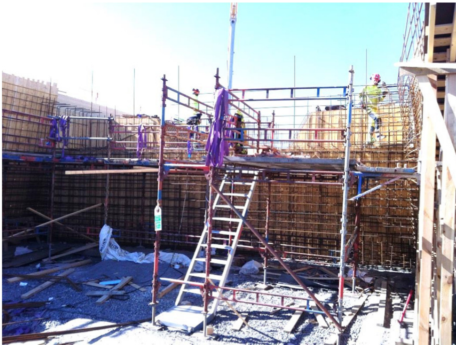
Figure 4.12 Fifty types of reinforcement are used in this bridge section.
