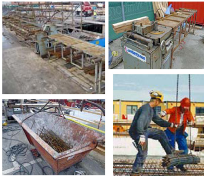
Figure 4.4 Reinforcement station at a site (Source: Persson, M., 2011).
