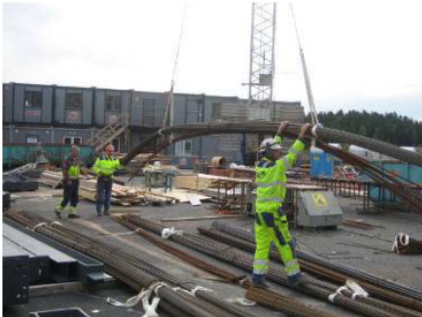
Figure 4.3 12m bars delivered to a site (Source: Caster, R. and Deuschl, G., 2007).
