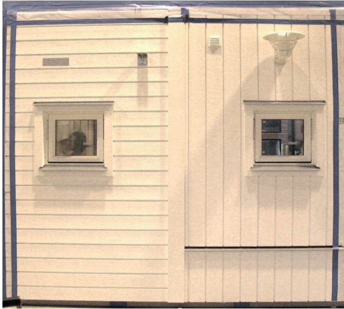
Figure 28. The two test items, manufacturer A, with horizontal and vertical wood panelling respectively.
