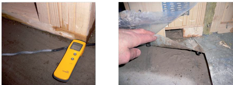
Figure 20. Observations from erection stage.
