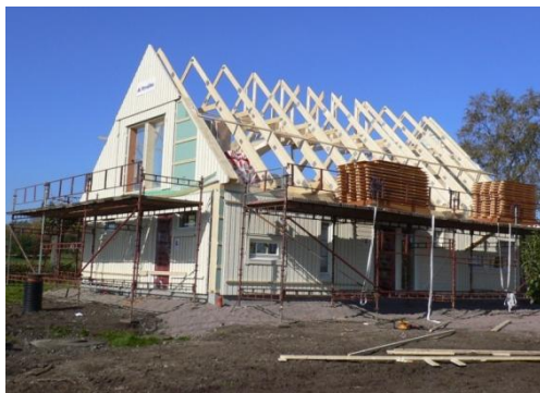
FIG 1. Erection of a detached house in progress.
