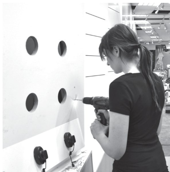
INSTALLATIONS FOR THE CELL PHONES ARE HIDDEN BEHIND THE WALL
