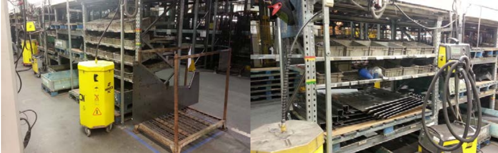
Figure 31. The Point-of-Use storage for the excavator and dumper stations
