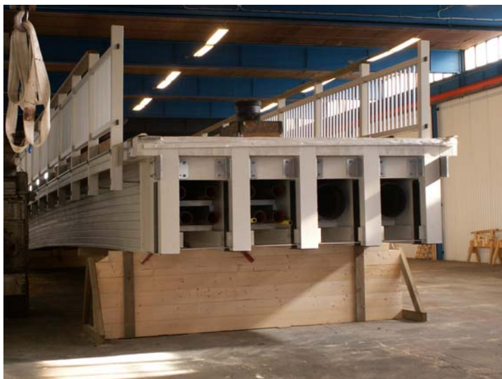
Figure 3.1 Assembling the whole bridge in the factory. (Moelven Töreboda)
