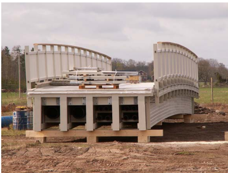
Figure 3.2 Transporting the prefabricated bridge into the site. (Moelven Töreboda)
