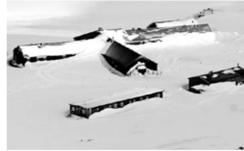
Today's station has a lot of problems with drifting snow
