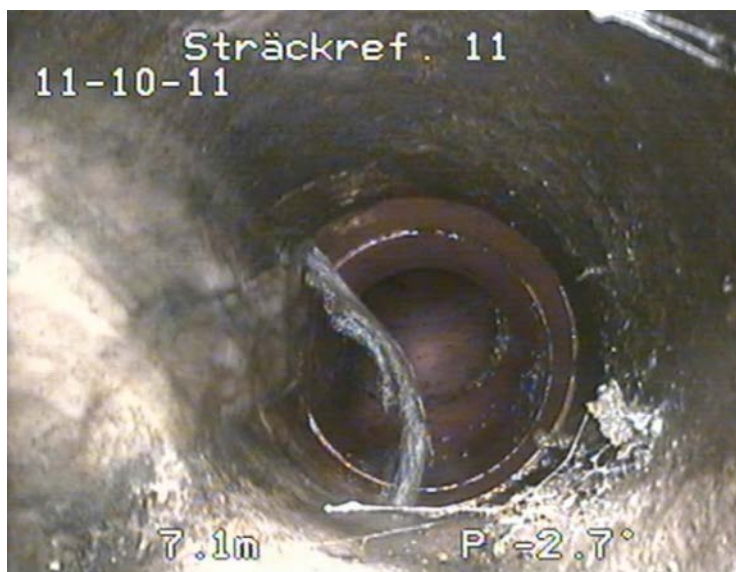
Figure 4: TV inspection showing a leak (Lunblad 2012)
