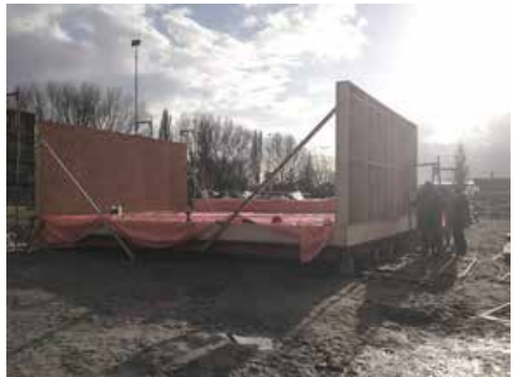
Concept Village CHIBB House under construction
