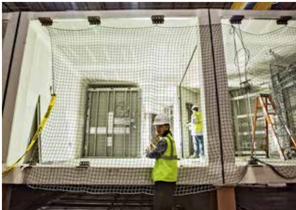
Fitting units out and together (Photo: Joel Arbaje, www.fastcoexist.com)
