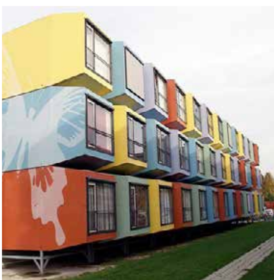
Constructed August 2004, (234 units) De Uithof Utrecht, student housing (nennyq.blogspot.com)
