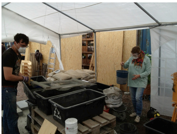
Figure 22: Sigurjónsson, Ásgeir (2013) Powderizing Gothenburg clay inside the mixing tent
