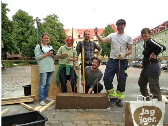
Figure 36: Sigurjónsson, Ásgeir (2013). First rammed section.
