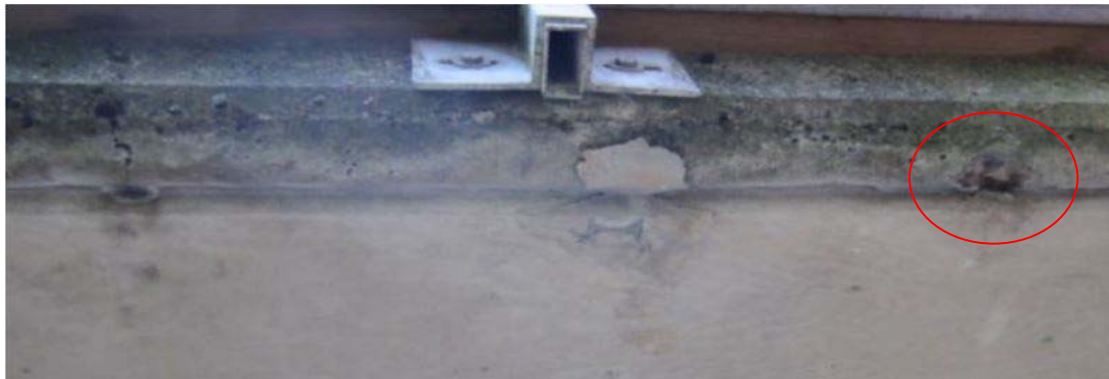
Figure 51 Corrosion crack found on the underside of a balcony
