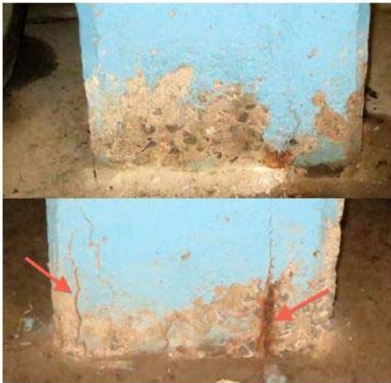
Figure 41 Column, located in the upper level, showing rust stains and corrosion cracks.
