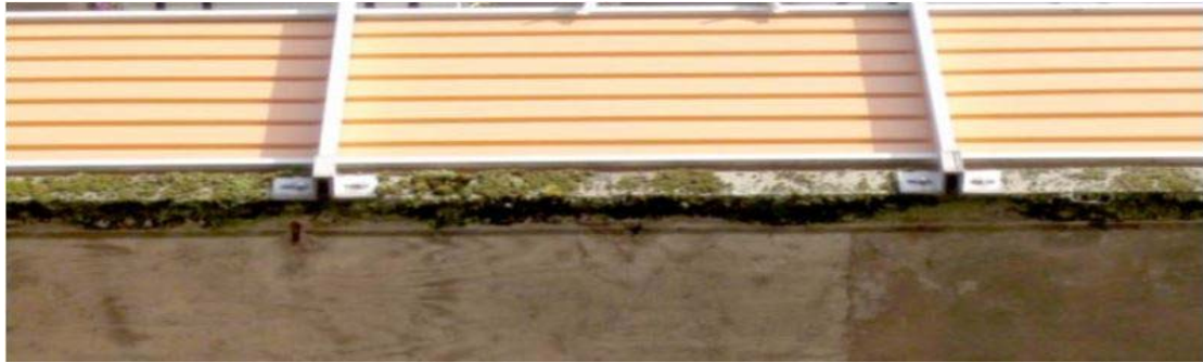
Figure 50 Image showing the construction of the balcony plates
