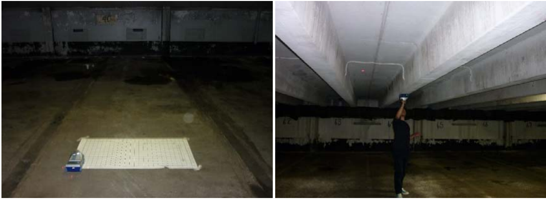
Figure 60 Onsite images of the floor element
