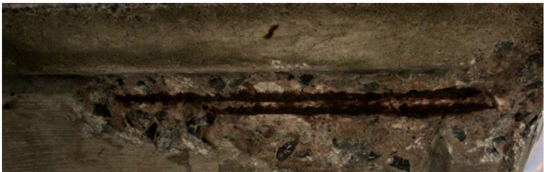
Figure 52 Corroded rebar on the underside of a balcony at Ivargårdsgatan
