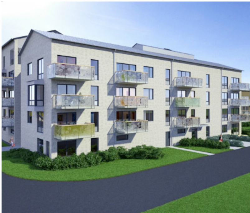
Figure 3.1. Example of how a house for which NCC Technical Platforms have been used can look like (Bostäder Tölöbergs Terrass etapp 1 , 2008-2014)
