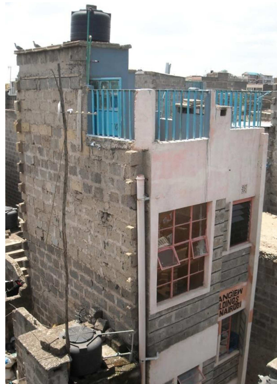
Figure 4.2 Completed 3-storey house.
