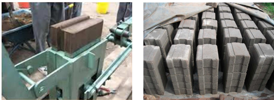
Figure 3.4 Left: freshly moulded ISSB ejected from block press. Source: Makiga Engineering (2010). Right: ISSBs stacked for curing/drying after moulding. Photo: author.
