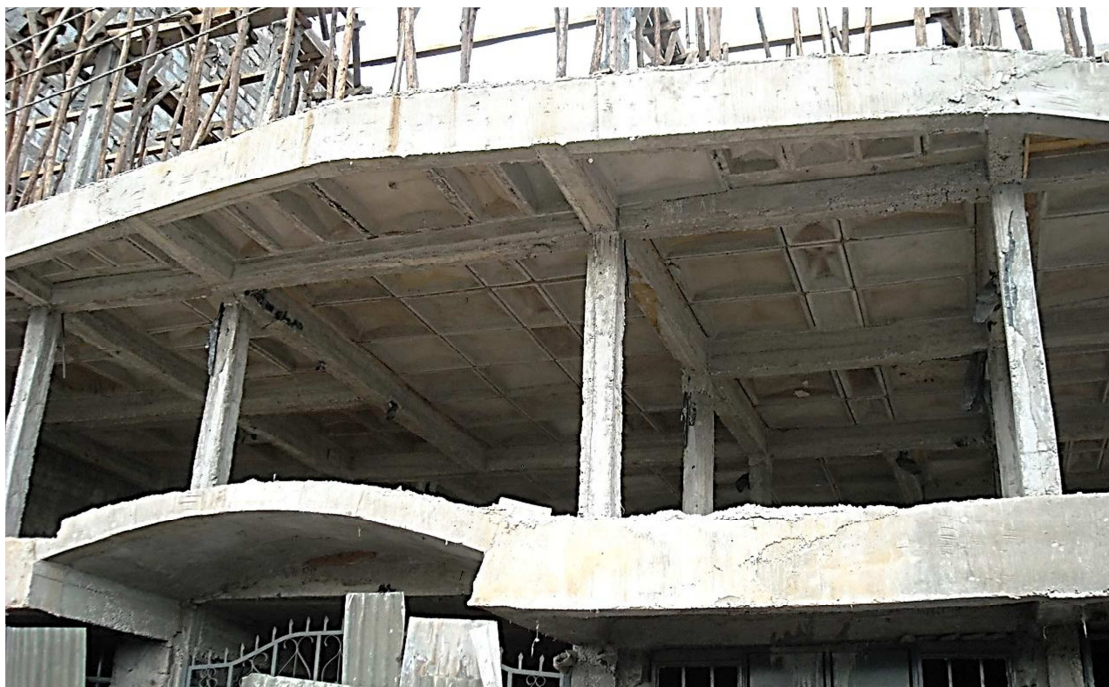
Figure 3.5 Multi-storey construction using waffle slab floor design: waffles supported by beams, reinforced concrete layer on top and reinforcement members between the slabs. Photo: author.
