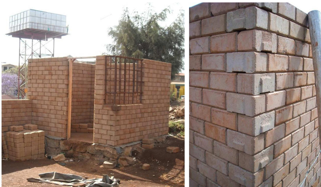
Figure 3.1 Left: demonstration building of ISSBs. Right: close-up showing block assembly. Photos: author.
