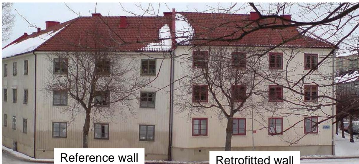
Figure 4.1. The three story county governor's house from 1930 chosen for the field study. The right part of the façade was retrofitted with vacuum insulation panels while the left part only had the wooden cover boards replaced and worked as reference wall (FIG 1 in Paper III).
