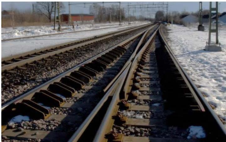
Figure 3. Overview of crossing panel from the rear of the turnout including a fixed crossing and check rails
