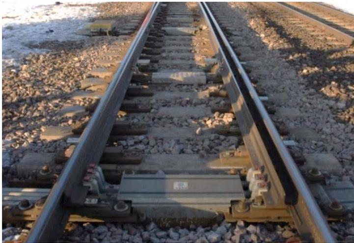
Figure 2. Overview of switch panel from the front of the turnout including switch rails and switching machines
