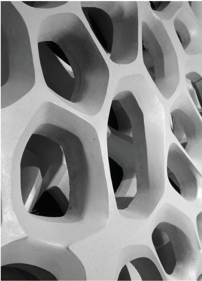
Fig. 25, "Cocoon Club", panellised concrete wall, design by 3deluxe, development of concrete elements by Villa Rocca
