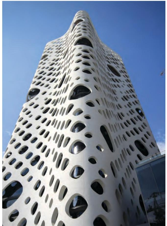
Fig. 23, "O-14", office tower in Dubai, external reinforced concrete structure, Reiser & Umemoto
