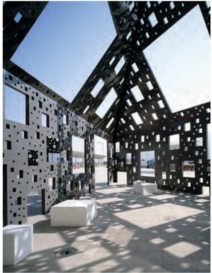
Fig. 28, "Shin Yatsushiro Monument", pre-cast walls and cast in place roof, 7cm thick glass fibre-reinforced concrete, Kumiko Inui
