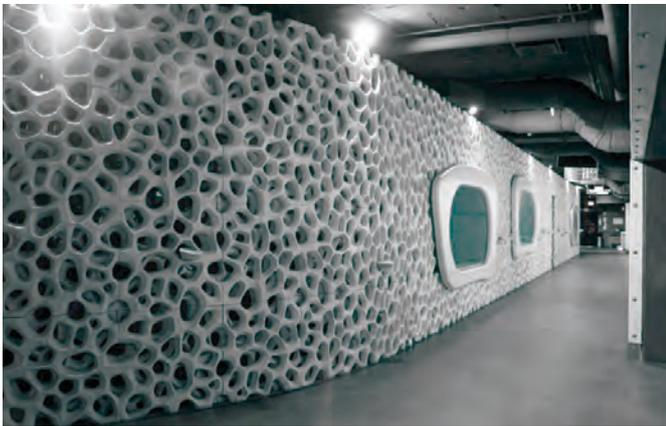
Fig. 26, "Cocoon Club", panellised concrete wall, design by 3deluxe, development of concrete elements by Villa Rocca
