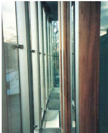
Figure 19 Typical shaft-box double-skin facade [Oesterle et al., 2001 p. 19]
