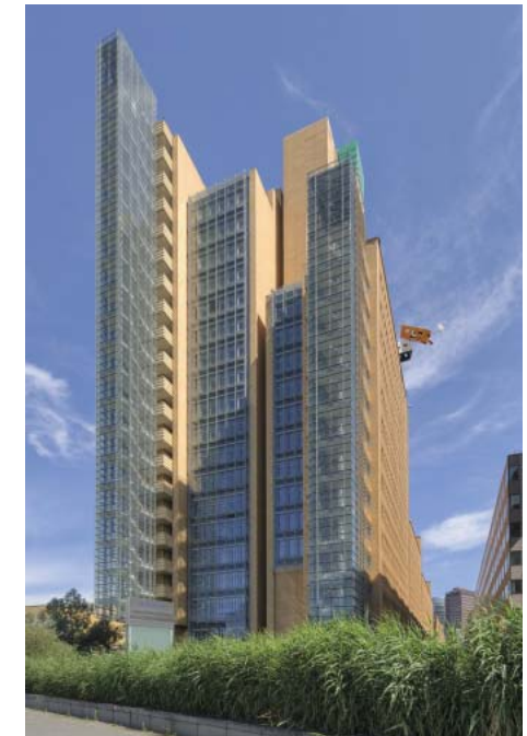
Figure 14 Debis HQ, R. Piano, Germany
