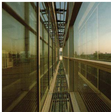
Figure 23 Multistorey facade with gratings for maintenance, Victoria Ensemble building, Germany [source: http://gaia.lbl.gov/hpbf/casest_m.htm ]
