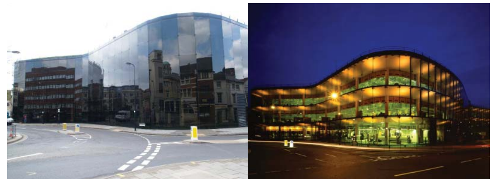
Figure 46 Willis and Faber Building, Ipswich, UK, Norman Foster
