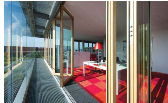
Figure 21 Corridor facade with totally operable inner casements [source: continuingeducation.construction.com]
