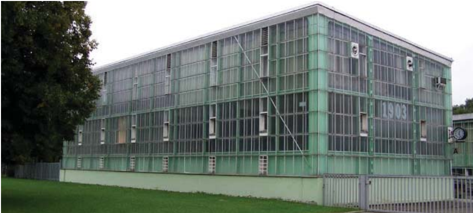
Figure 7 : Margarete Steiff AG factory today [source: www.facadesconfidential.blogspot.se]
