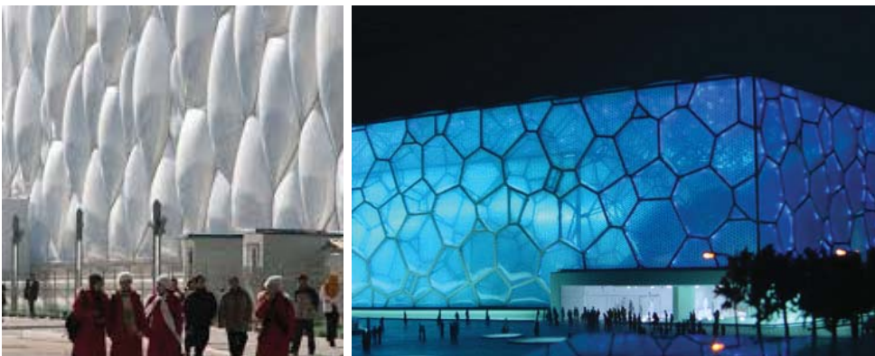
Figure 32 Water Cube (Olympic Swimming center), Beijing, China, Herzog and De Meuron
