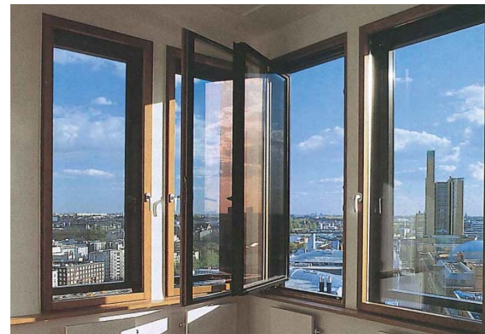
Figure 17 Box window facade [Oesterle et al., 2001 p.15]
