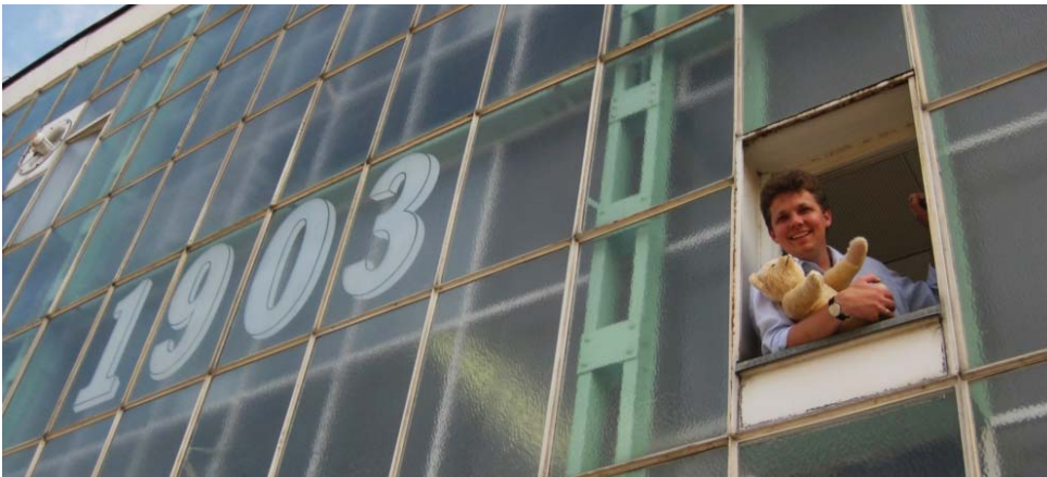
Figure 8 : Margarete Steiff AG factory today, The pillars inside the intermediate space, the floor and the ceilings create the box-type window facade [source: www.facadesconfidential.blogspot.se]
