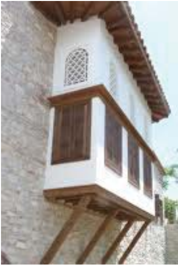
Figure 4 : Hayiati with wooden shutters [source: personal archive]
