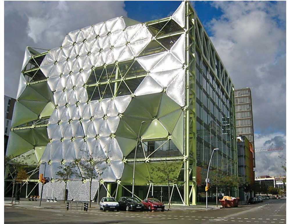
Figure 33 Media-TIC, Barcelona, Spain, Architect Enric Ruiz-Geli (Cloud 9)
