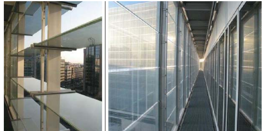
Figure 24 Typical louver naturally ventilated double-skin facade [BBRI, 2004, p.12]
