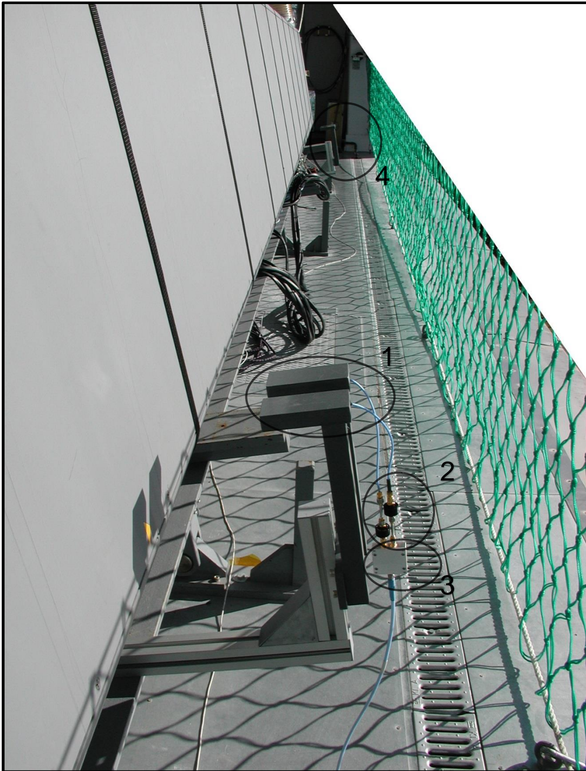
Figure 13: Close up of sensor mountings. 1 – Receiving antenna pair in plastic encasing. 2 – Attenuators protecting the power combiner. 3 – Power combiner. 4 – Second sensor mounting.
