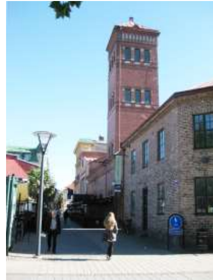
Figure 1 Fattighuset at the corner, next to the fire brigade's hose tower.
