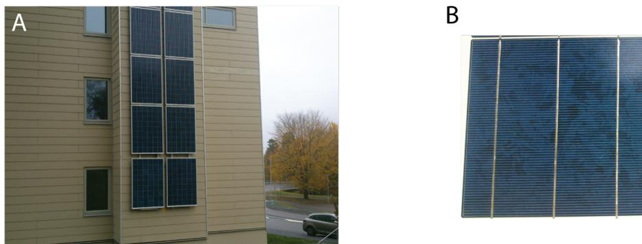
**Figure 2.1.** (A) A module made of polycrystalline Si solar cells, mounted on a wall of a residential building in Göteborg, close to where the author lives. (B) One of the cells in the module.
