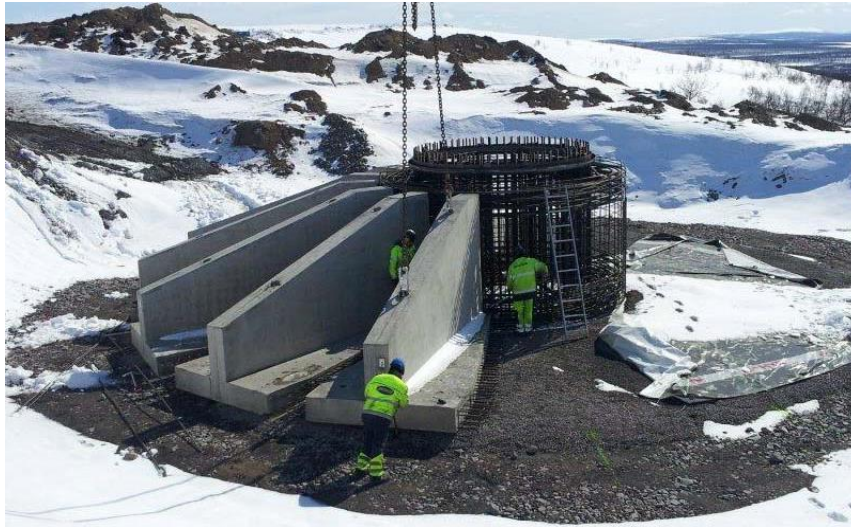
Figure 4.1: Assembling of the foundation, the elements are attaching to the reinforcement basket. (Sjisjka vind 2013).
