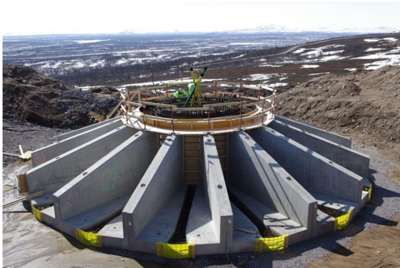
Figure 4.3: The elements and the moulds, placed at the correct position before casting of fresh concrete can start. (Sjisjka vind 2013).
