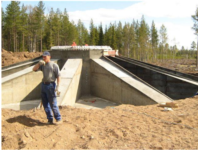
Figure 4.4: Star foundation at Bondön, onsite cast at this specific site. (Hägström 2013).
