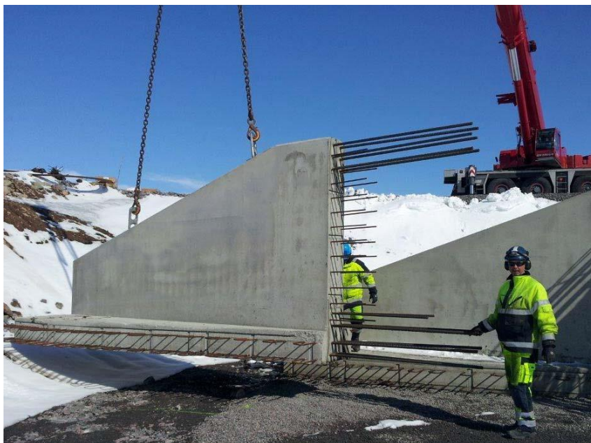
Figure 4.2: One element for the foundation at Sjisjka, which here is lifting on place. Here is also the protruding reinforcement visible. (Sjisjka vind 2013).
