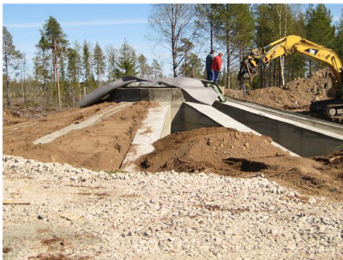
Figure 4.5: The star foundations are covered with excavated soil in order to increase the self-weight. (Hägström 2013).
